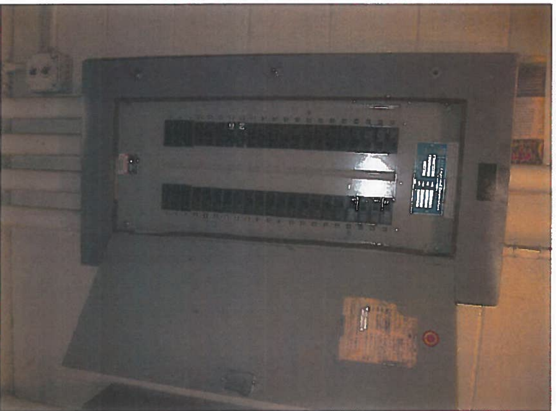
EXISTING PANEL "LP-F"
