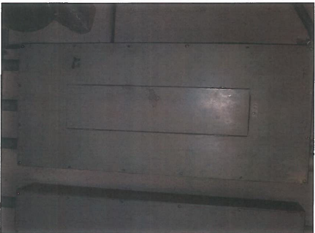
EXISTING PANEL "LP-F"
